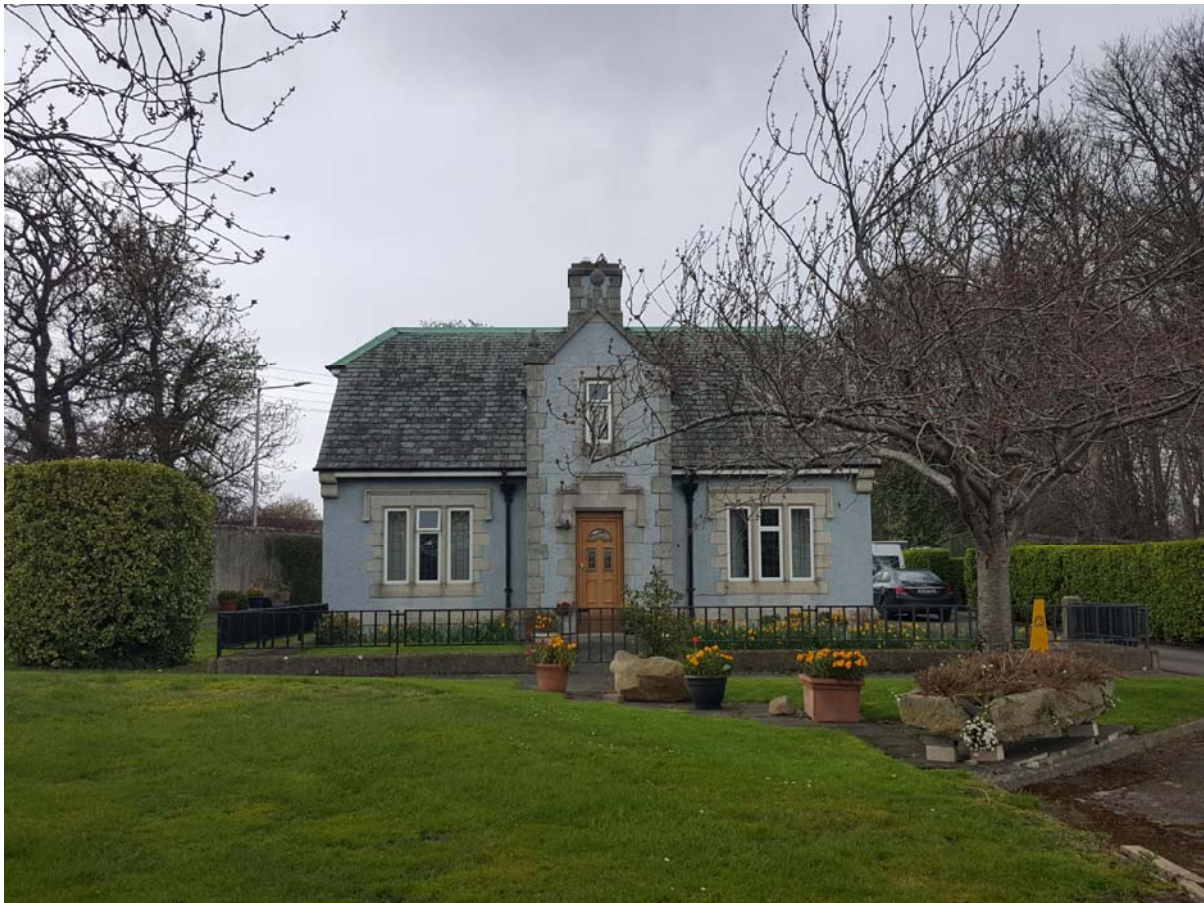
Image 13.57: Byrne's c.1925 gate lodge contributes to the architectural integrity of the demesne, despite its later provenance. It effects both an Arts & Crafts as well as a Gothic idiom that makes it a creative but sympathetic part of the landscape (RPS ref. 1845; NIAH ref. 60260148).
