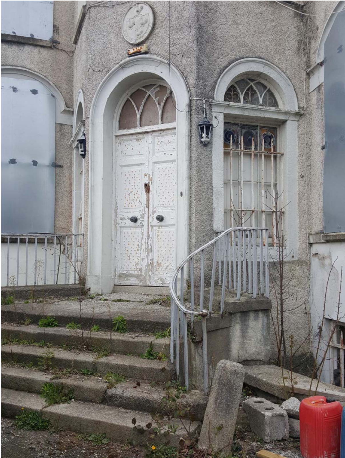
Image 13.50: The entrance, set to the western half of the building, is at a lower level than the areas to the east, owing to Morrison's extensions. Note the panellled shutters seen to the interior.
