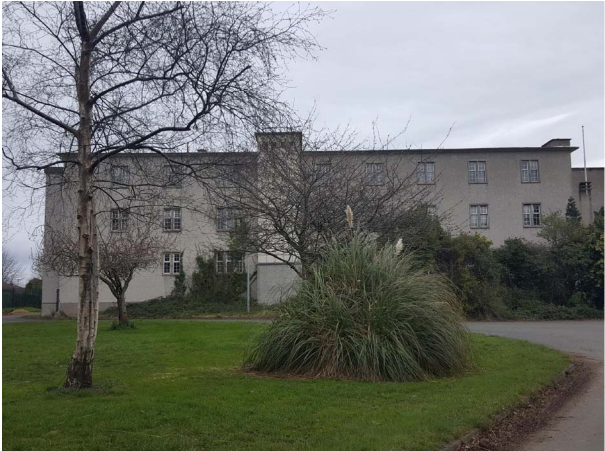
Image 13.27: This fork of the entry drive that turns northward in front of the 1950s block once lead to the stable yard.
