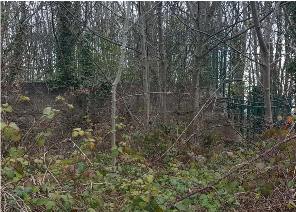
Image 13.34: To the north of the castle, a portion of the original field boundary wall survives. This is outside the development boundary.
