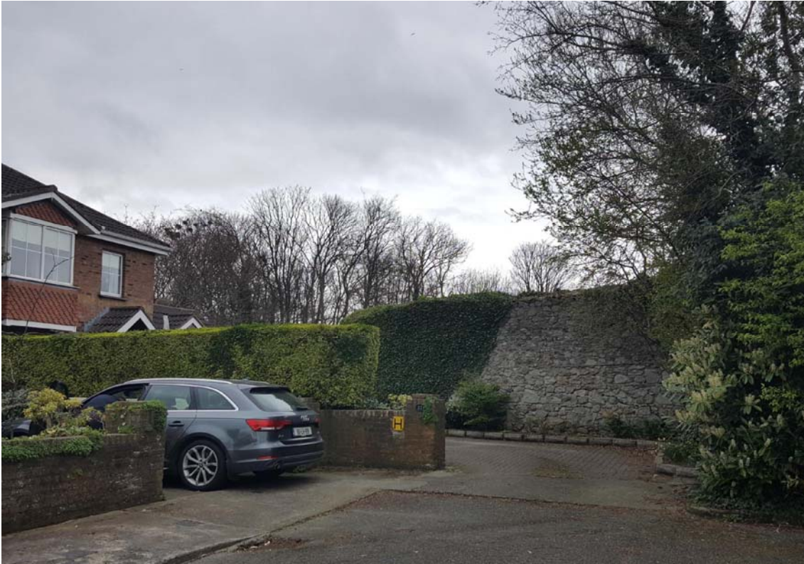
Image 13.35: Part of the stable yard boundary wall survives adjacent to Castle Farm housing estate. This is outside the development boundary.
