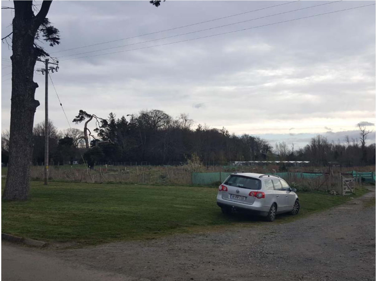
Image 13.41: The depot (background, above) is situated between the planted woodland and the ornamental pond and impacts the setting of both features.
