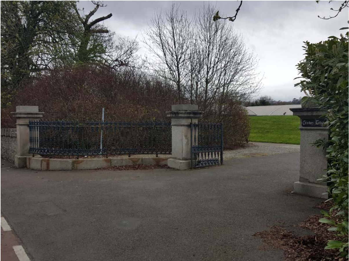
Image 13.60: The cut granite piers and cast-iron railings located just to the north of the gate lodge and on the western side of Dublin Road mark the later entrance to Crinken Lodge (NIAH ref. 60260151).
