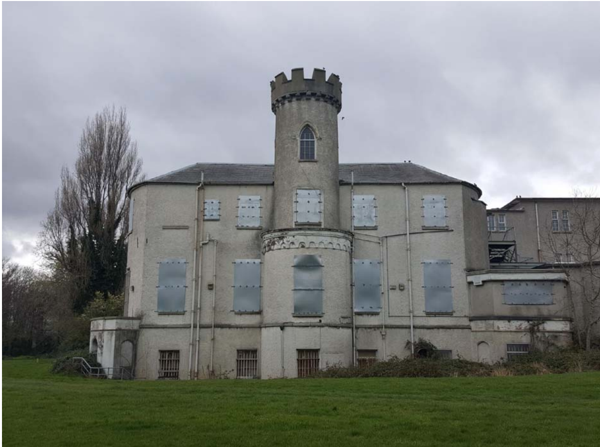
Image 13.53: The rear (north-east) elevation of the castle more readily presents the original, double bow-ended house, with the central turrets being added by Morrison.
