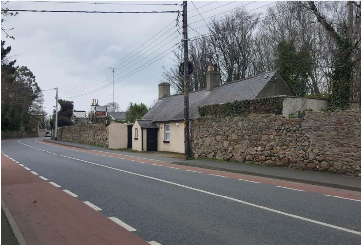
Image 13.62: Between the c.1925 gate lodge and Crinken Cottage stands a small cottage that was not recorded by the NIAH nor placed on the Record of Protected Structures, but it does appear as early as the Ordnance Survey of 1837. Its roof weatherings and windows have been replaced, but its form, siting and immediate context are retained, thereby contributing to the historic character of the area.
